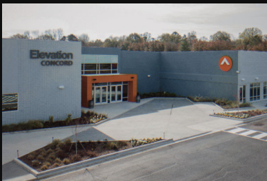
CONCORD Launch: October 20, 2013 New Building: June 28, 2020
